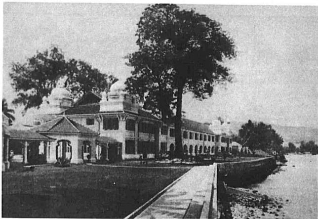
Eastern and Oriental Hotel, Penang, showing the Victory Annex, constructed in 1922. (Photo credit: 'Penang. The City and Suburbs in the Early Twentieth Century', Georgetown Printers, 1986.)
